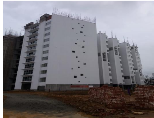
Ghatail Cantonment Senaneer Building
