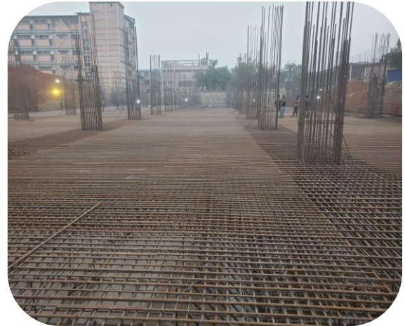
Renaissance Iconic Building
