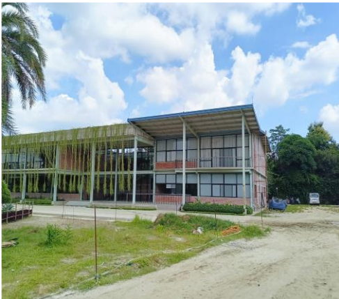
Renaissance Apparels Ltd. Annex Building
