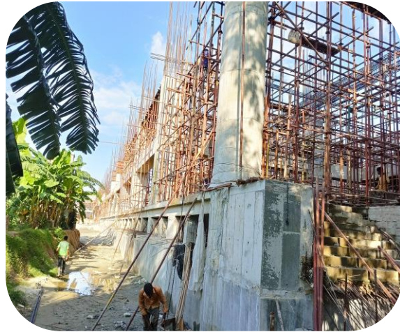
Renaissance Iconic Building
