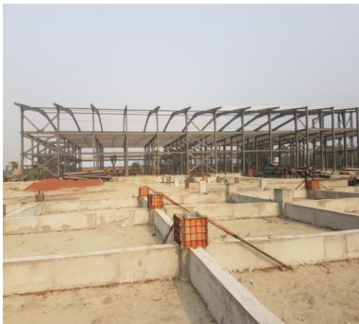
Renaissance Apparels Ltd. Annex Building
