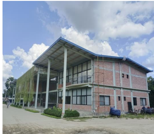
Renaissance Apparels Ltd. Annex Building
