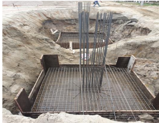
Renaissance Apparels Ltd. Annex Building
