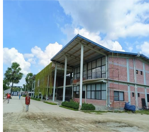
Renaissance Apparels Ltd. Annex Building
