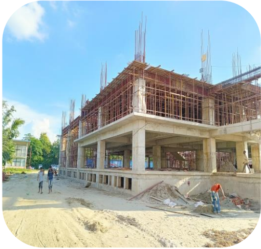
Renaissance Iconic Building
