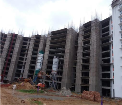
Ghatail Cantonment Senaneer Building
