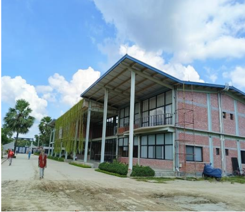
Renaissance Apparels Ltd. Annex Building
